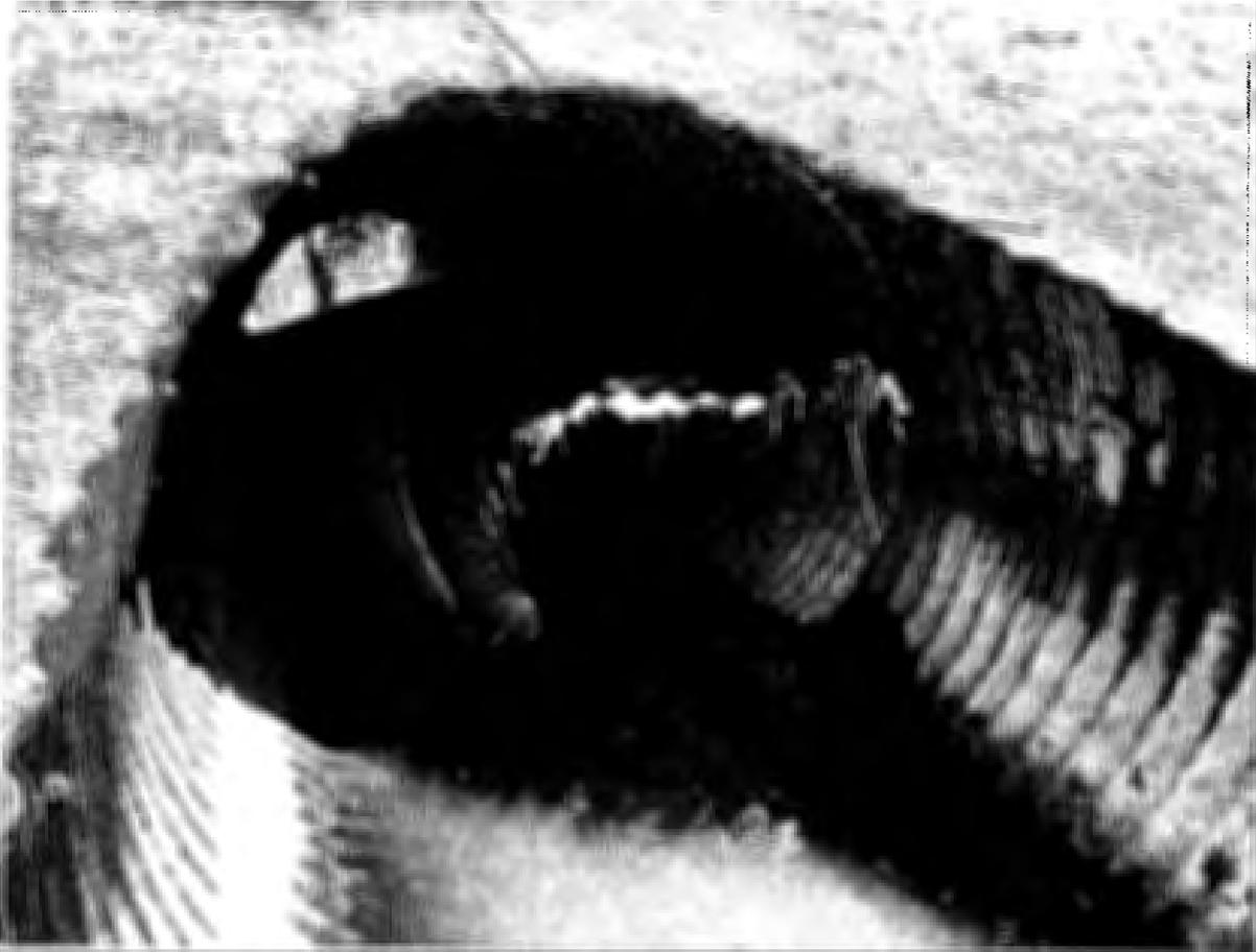
Our bridge technologist examined this culvert and noted that much of the granular backfill had washed out around this pipe, leaving about 20 feet of unsupported concrete deck. The crossing was immediately closed to all traffic.
